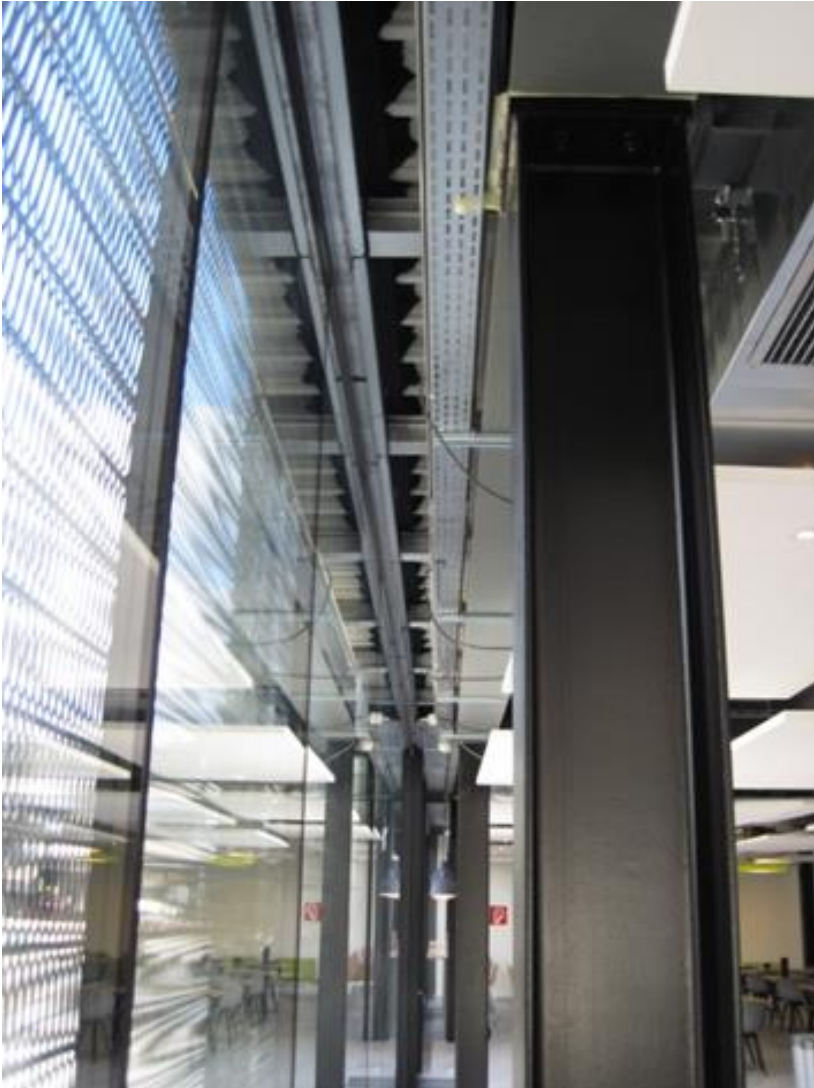
Detail of the glass façade.
