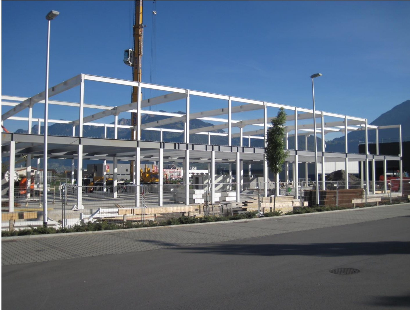
Shopping centre in Collombey
