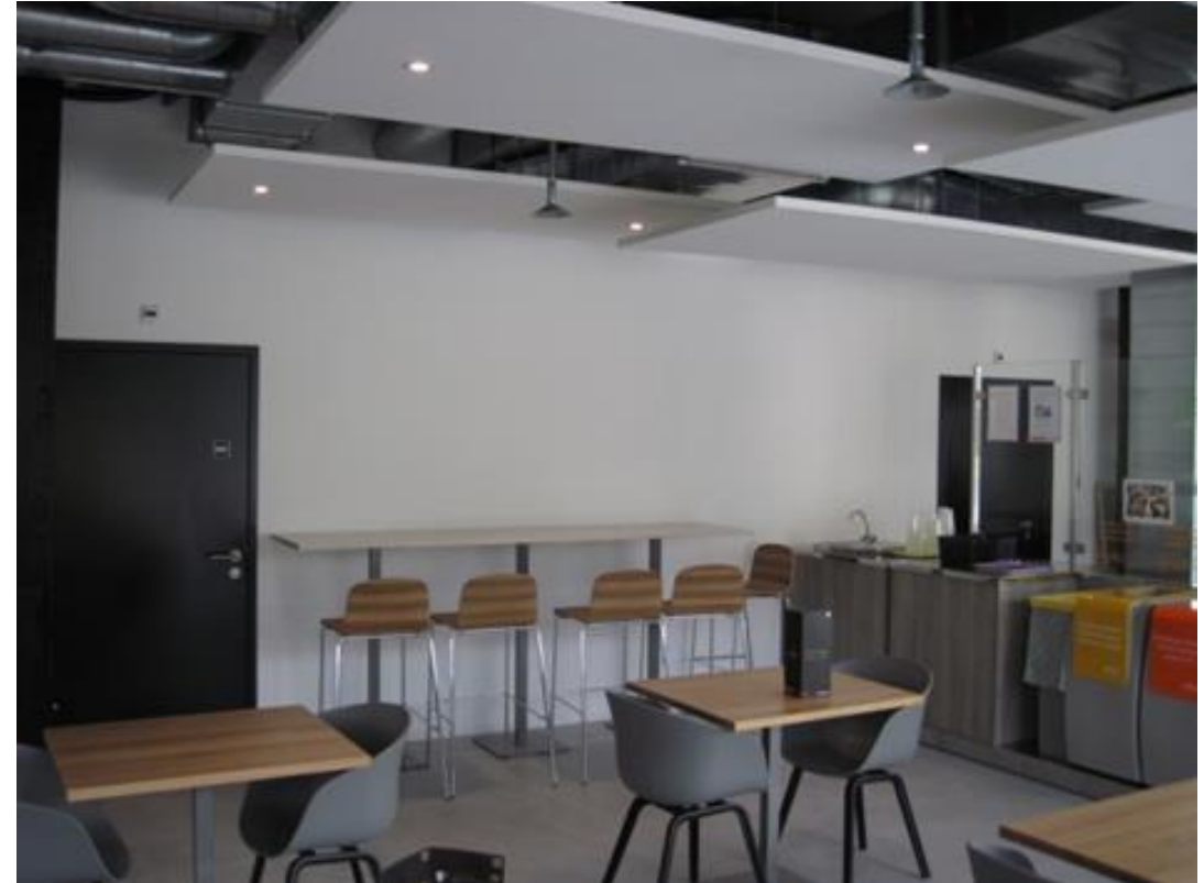
Partition wall between the restaurant, the back office and the toilets.
